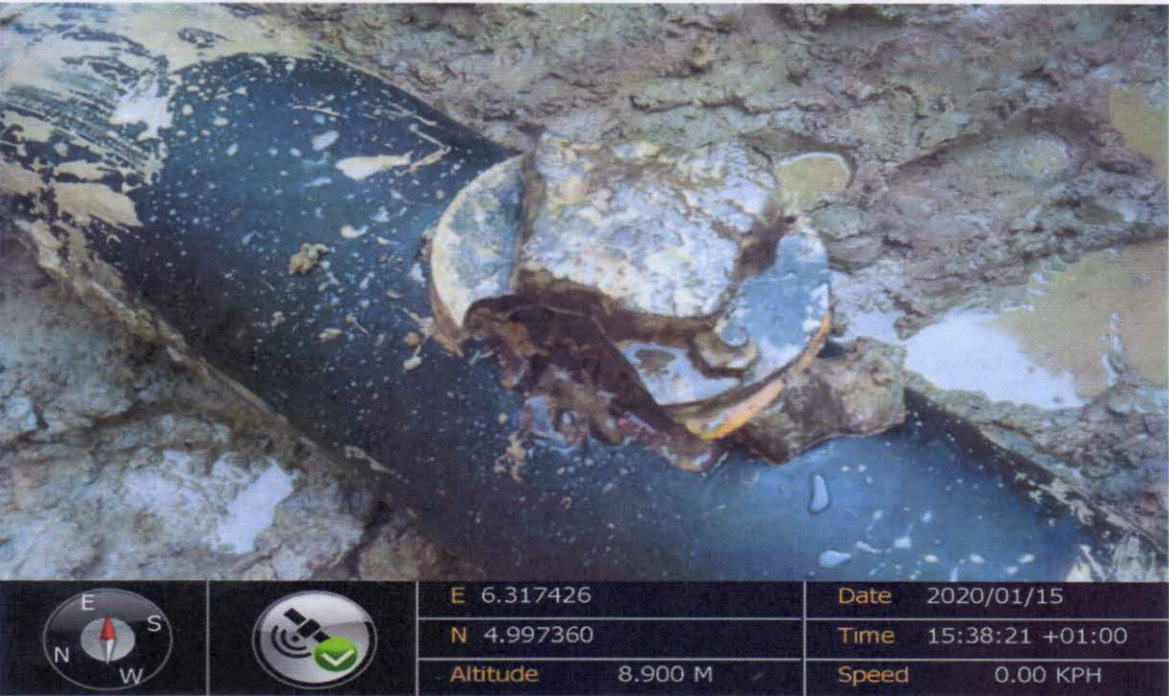
FIG. A: SHOWING A 3” FLANGE INSTALLED AT 12 O’ CLOCK POSITION OF THE PIPELINE
